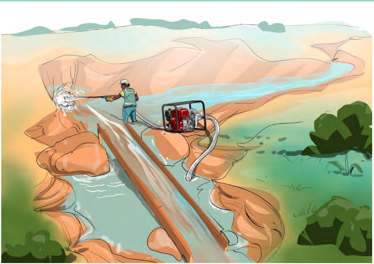
Image 30: Motor pump used to break loose ground.
