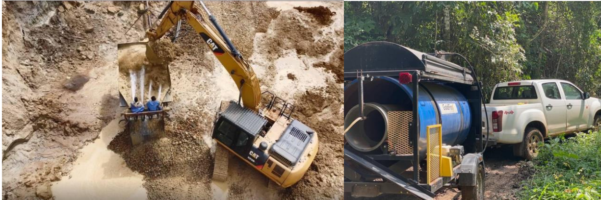
GoldFinX machinery and equipment investments; (left) excavator in action and (right) is a trommel wash plant intended for small batch testing (10 tonnes/hour)
