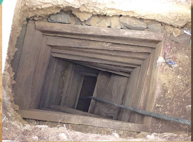
Well timbered shaft
